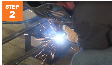
Weld angle iron supports.
