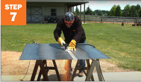
Cut 1/8" steel plate.
