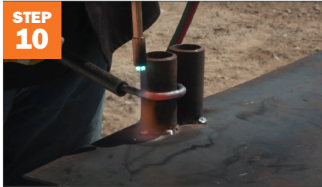
Heat and bend 3/8" rebar for tie down hooks.
