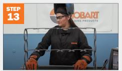
Place one piece of rebar in the center of the bottom horseshoes.
