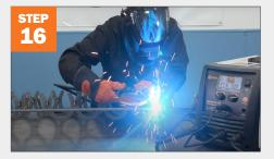
Weld all the way around both sides of the rebar.
