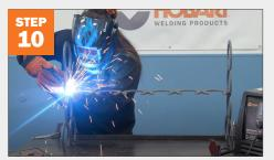
Complete the weld on each side, for extra support weld underneath.
