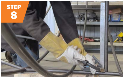
Mark and place seat support bars, and weld.
