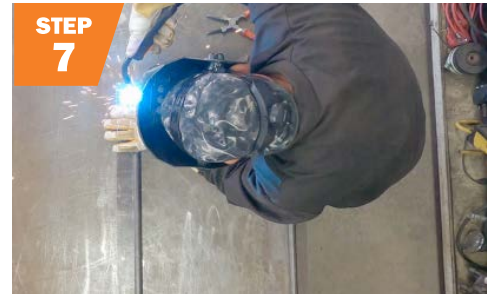
Measure and cut pipe tubing for bench seat, and weld.
