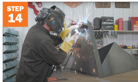
Weld the legs to the bottom.
